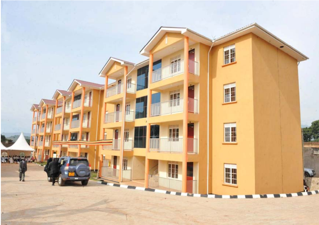
Staff apartments at Mbale Hospital
