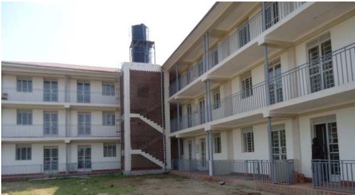
Staff accommodation: Kabale hospital Nurses hostel almost complete.
